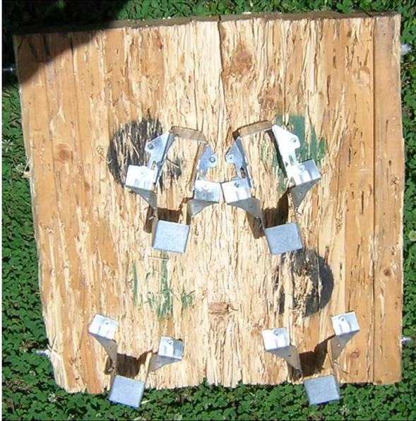
Backside showing joist hangers. Legs will go out bottom of picture.
