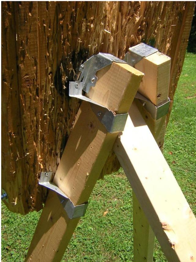
Closeup of back to show how joists hangers are positioned and legs inserted.
